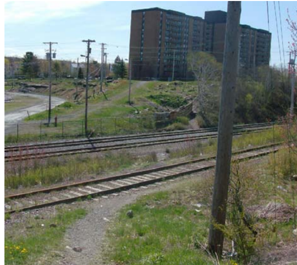
Figure 3-8: Superstore Rail Crossing
