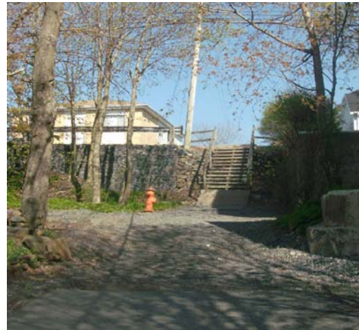
Figure 3-4: Douglas Drive Stairway
